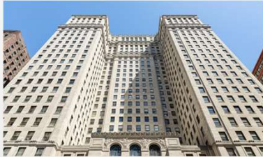
123 S. Broad St. Units 1 & 2 $4.1MM financing Energy & Water Measures
