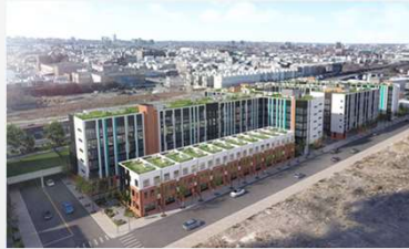
Somerset Station $17.9MM new construction financing Energy & Water Measures
